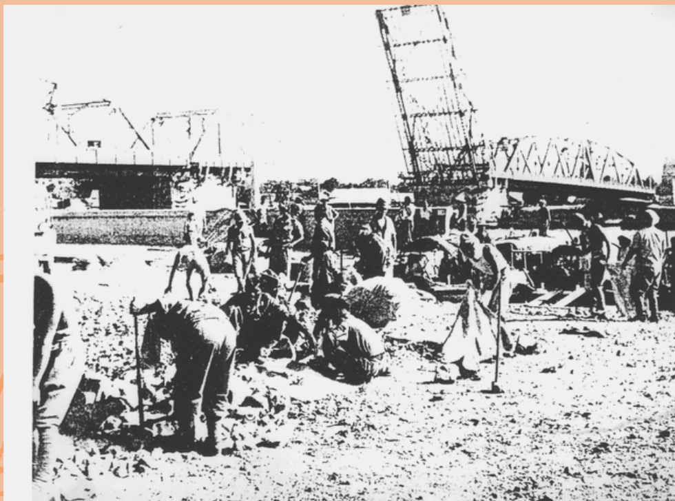
Former Japanese soldiers repairing Bangkok bridge end 1945, under the command of Sapper Roy Hudson.
